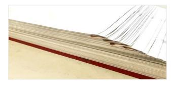
If construction site condition is allowed, installer need to clean the subfloor and pave an effective damp proof membrane. Open flooring rolls package until fully spread, stack the pieces in one pile till the edge of flooring is completely flat.
